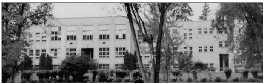
Vernon High School in Polson Park, 1954. It was demolished in 1998.
